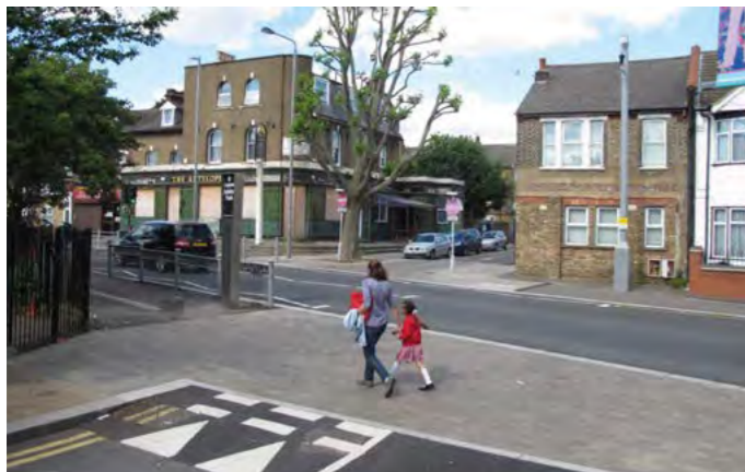
Example of continuous footway
