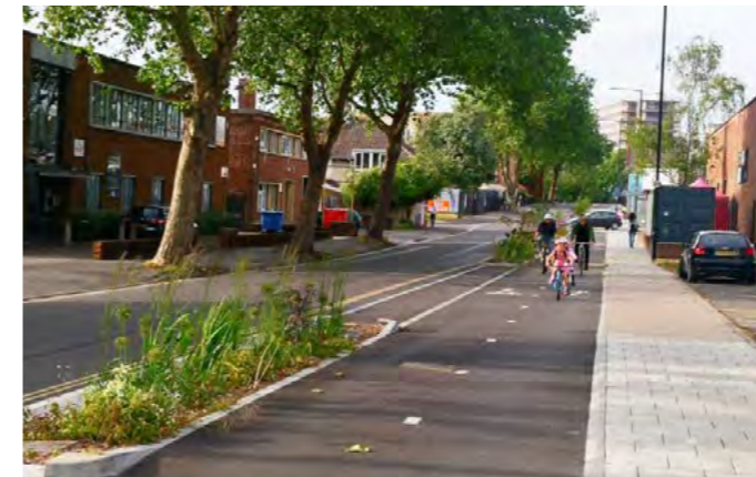
Existing Whitehouse Street cycle track.
